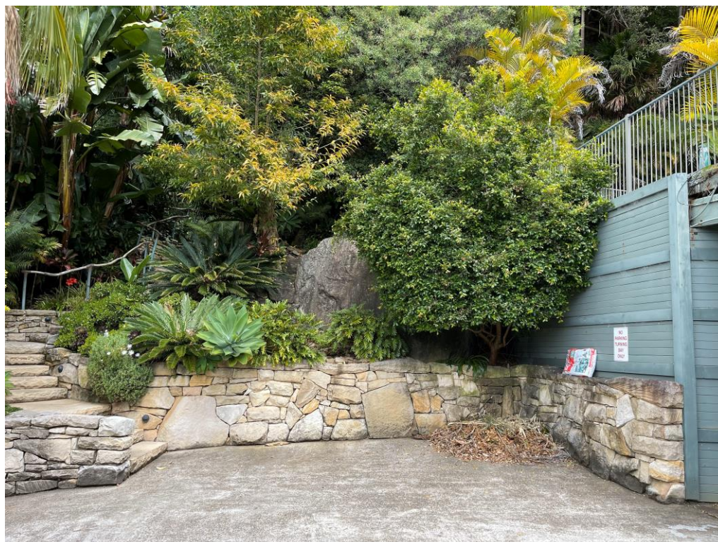
Fig 7: View of the proposed garage area, looking south-west
