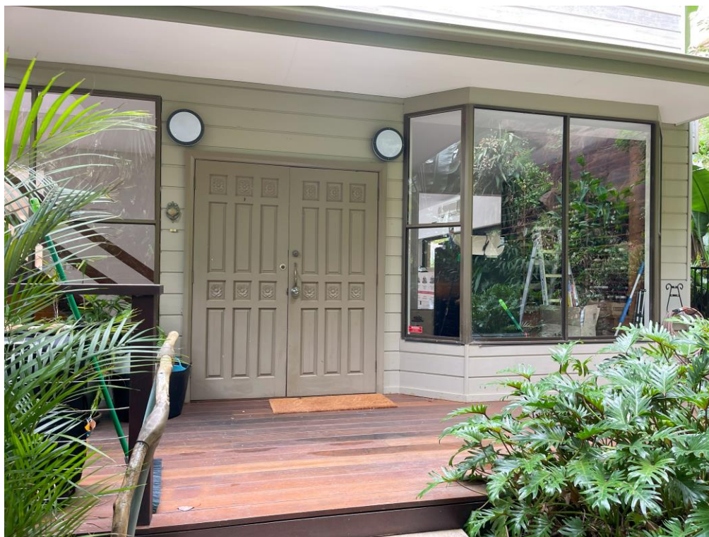
Fig 9: View of the existing front door and entry deck, looking south-east
