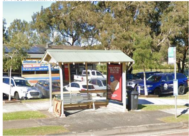
Figure 10 Existing C4 Bus Stop and Shelter on Pittwater Road, in front of 3 Arnott Crescent, Warriewood
