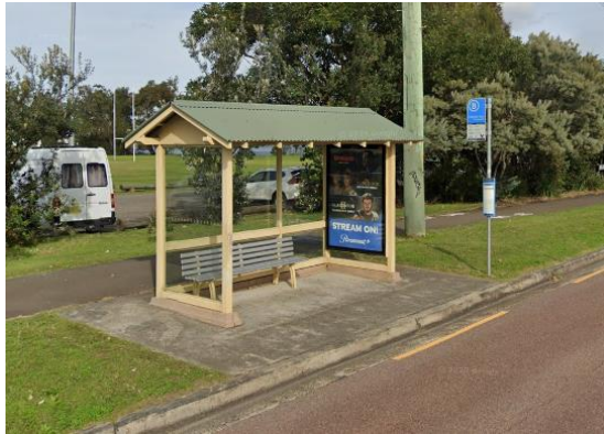
Figure 7 Existing C1 Bus Stop and Shelter on Pittwater Road, opposite of 1525 Pittwater Road, North Narrabeen
