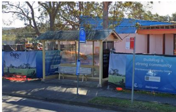
Figure 11 Existing C5 Bus Stop and Shelter on Jacksons Road, in front of Warriewood Community Centre, Warriewood.
