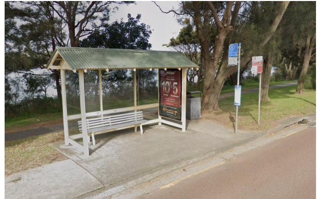
Figure 8 Existing C2 Bus Stop and Shelter on Pittwater Road, opposite of 1483 Pittwater Road, North Narrabeen
