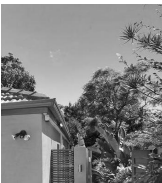
2. STREETVIEW - BUILDING TO BE RETAINED
