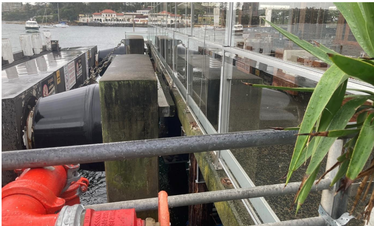
Figure 7: View of an example of the retractable glazed balustrade proposed for the site. This balustrade is outside the Hugos Manly restaurant on the western side of the wharf.
