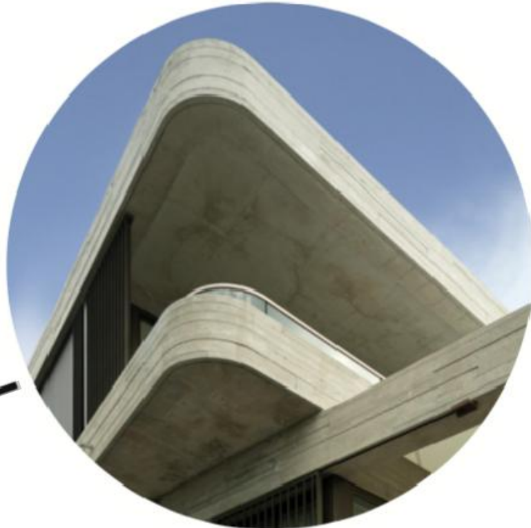
OFF FORM CONCRETE
