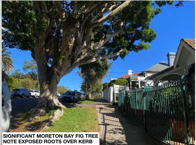
SIGNIFICANT MORETON BAY FIG TREE NOTE EXPOSED ROOTS AT DRIVEWAY CROSSING AND OVER KERB
