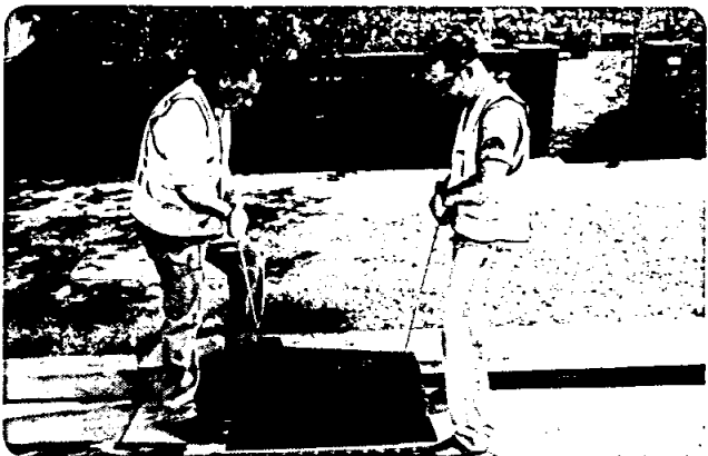
Photo 9 Lift grate above the support frame
