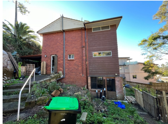
Photo 2: Southern side of residence
