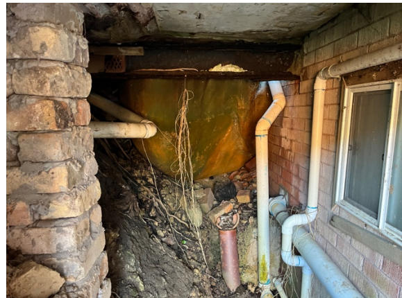
Photo 6: Sandstone boulder under the slab at the south-western corner of the house sits upon uncontrolled fill, sandy materials and brick pieces.
