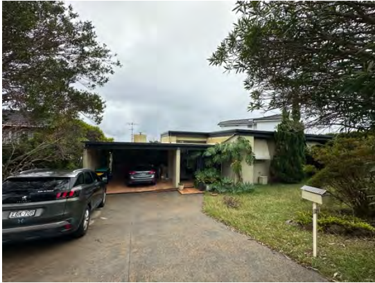
Photo 1: Site frontage, looking west.
