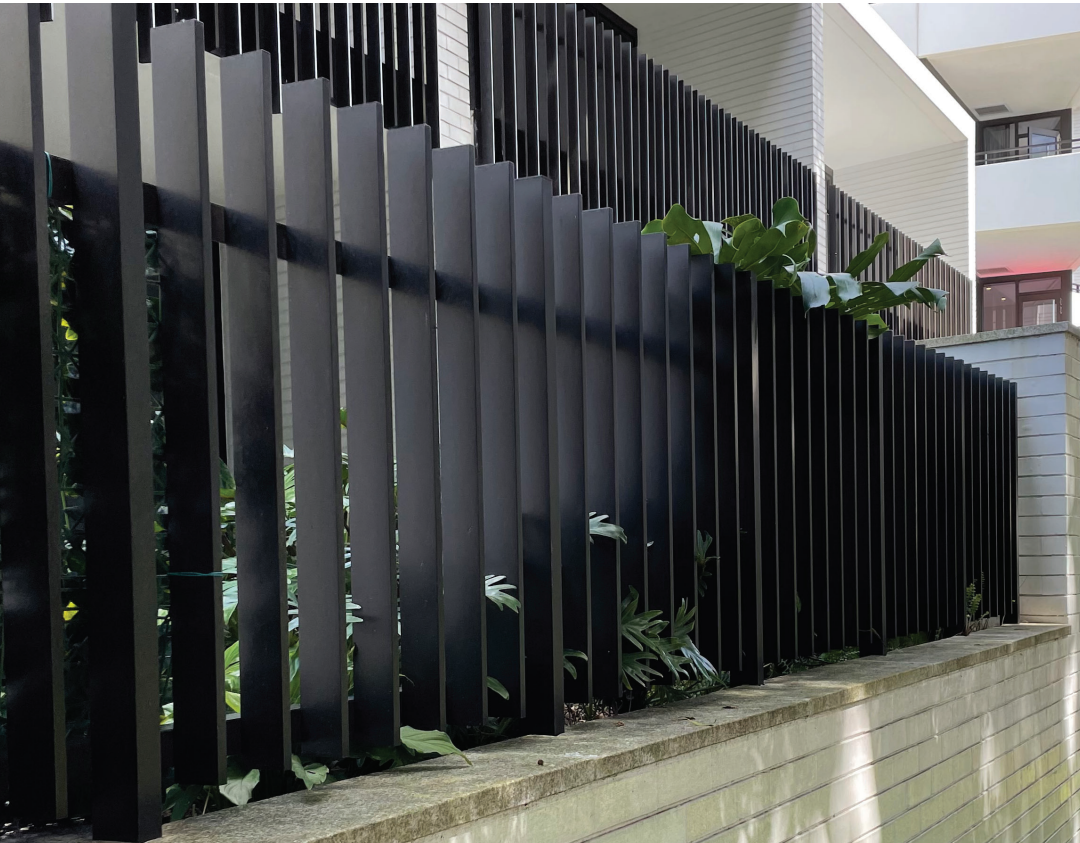
Fence Type 1 and 2: Metalwork fencing with vertical blades will match fencing used throughout the new development and provide an attractive and secure edge to the external spaces. Fence Type 1 is 1800mm height and will form the secure boundary to the external spaces. Fence Type 2 is 1000mm height and will form barriers between the external play spaces.
