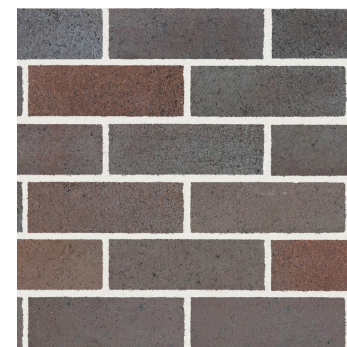
FACE BRICKWORK BRK2
