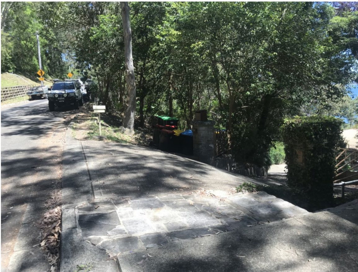
Existing accessway, noting excessive slope.
