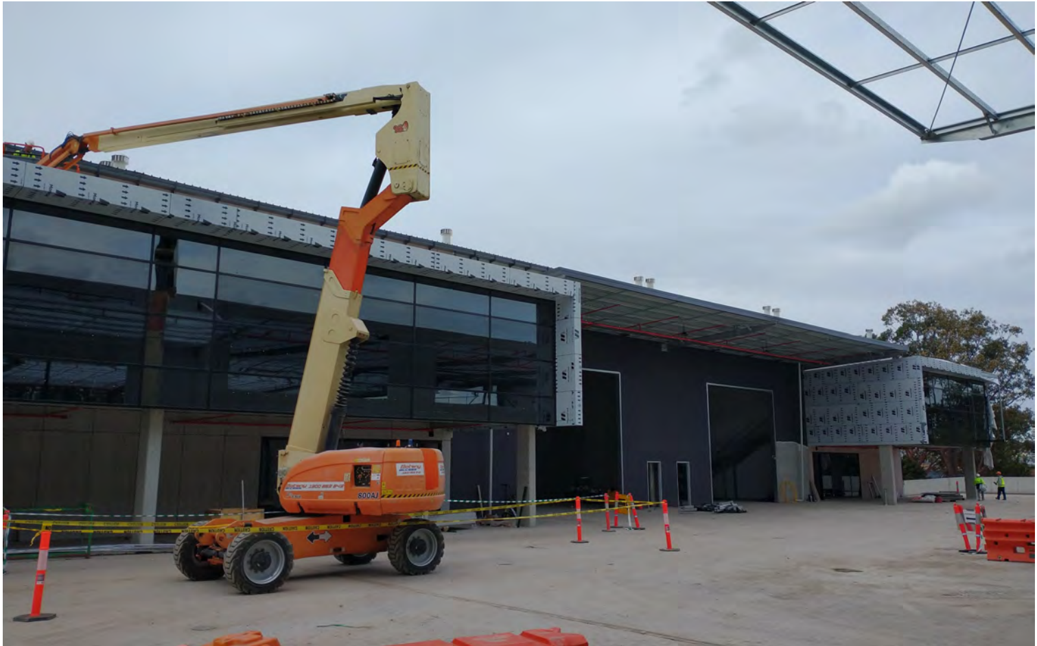
Photograph 1 (facing south-east): View of warehouse and driveway areas on Level 1. Note whirlybird ventilators for the SVVS outlet risers visible at the roof level.
