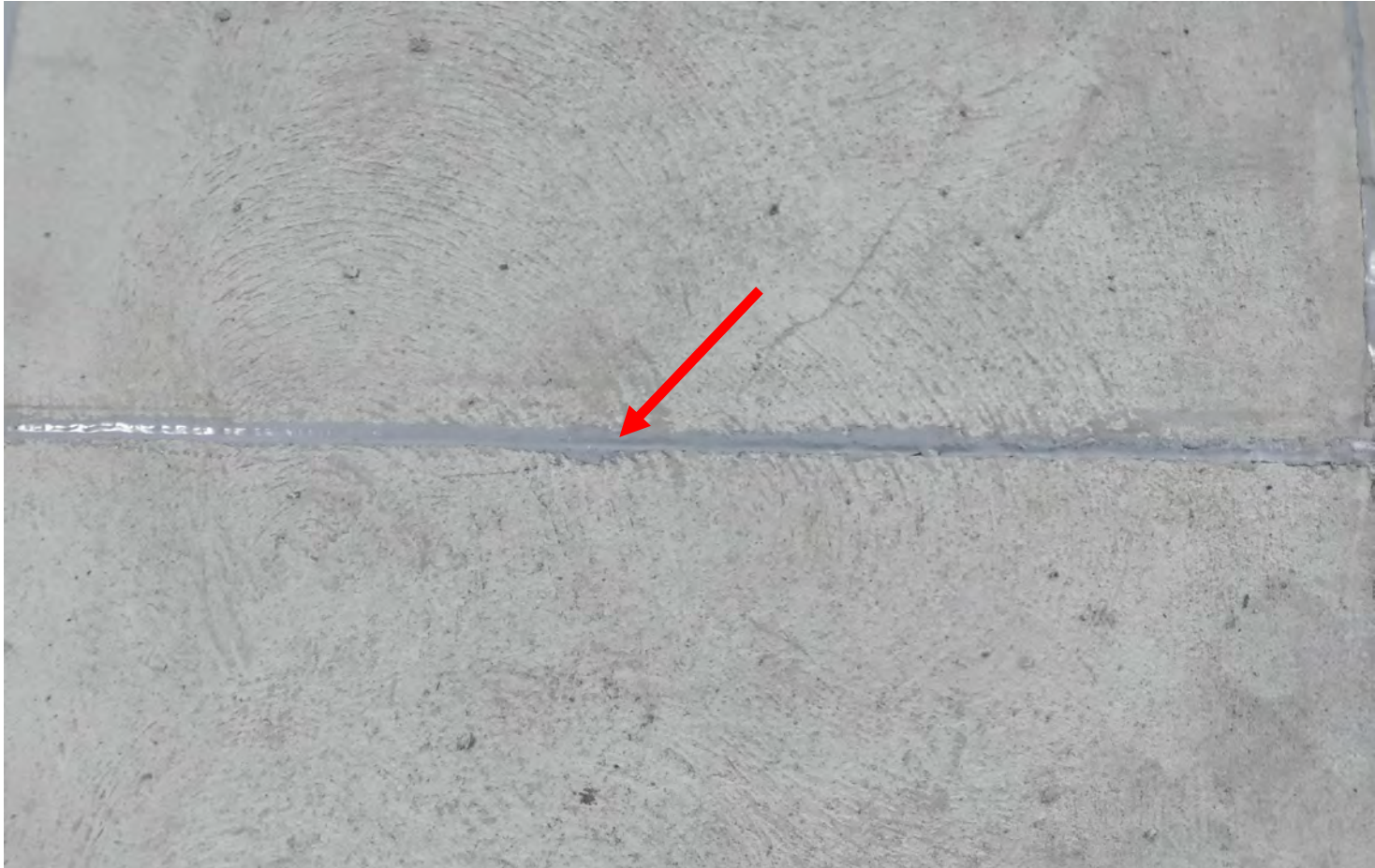
Photograph 10: View of typical caulking seam (red arrow) between expansion joints of the concrete floor and along the north wall at SSA#1. No cracks or evidence of shrinkage should be observed.
