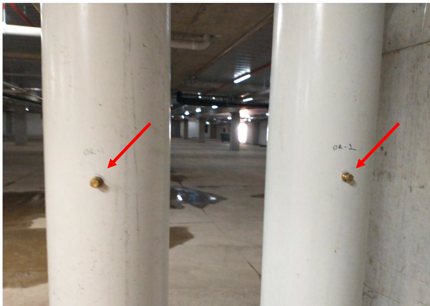
Photograph 8: View of typical brass sampling ports (red arrows) at the outlet risers (locations OR-1 and OR-2 shown).
