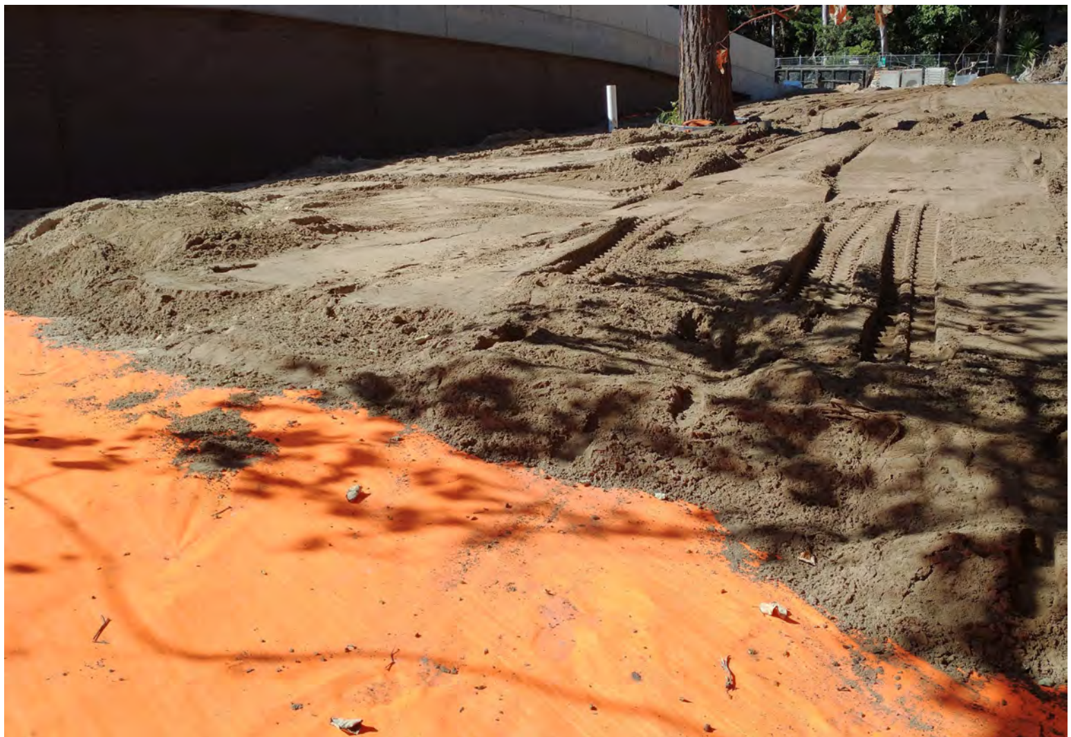
Photograph 2: View of orange marker layer during construction of capping.
