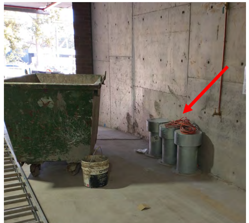
Photograph 3: View of three of four air inlet bollards (red arrow) at the entrance driveway on the lower level to the self-storage areas.
