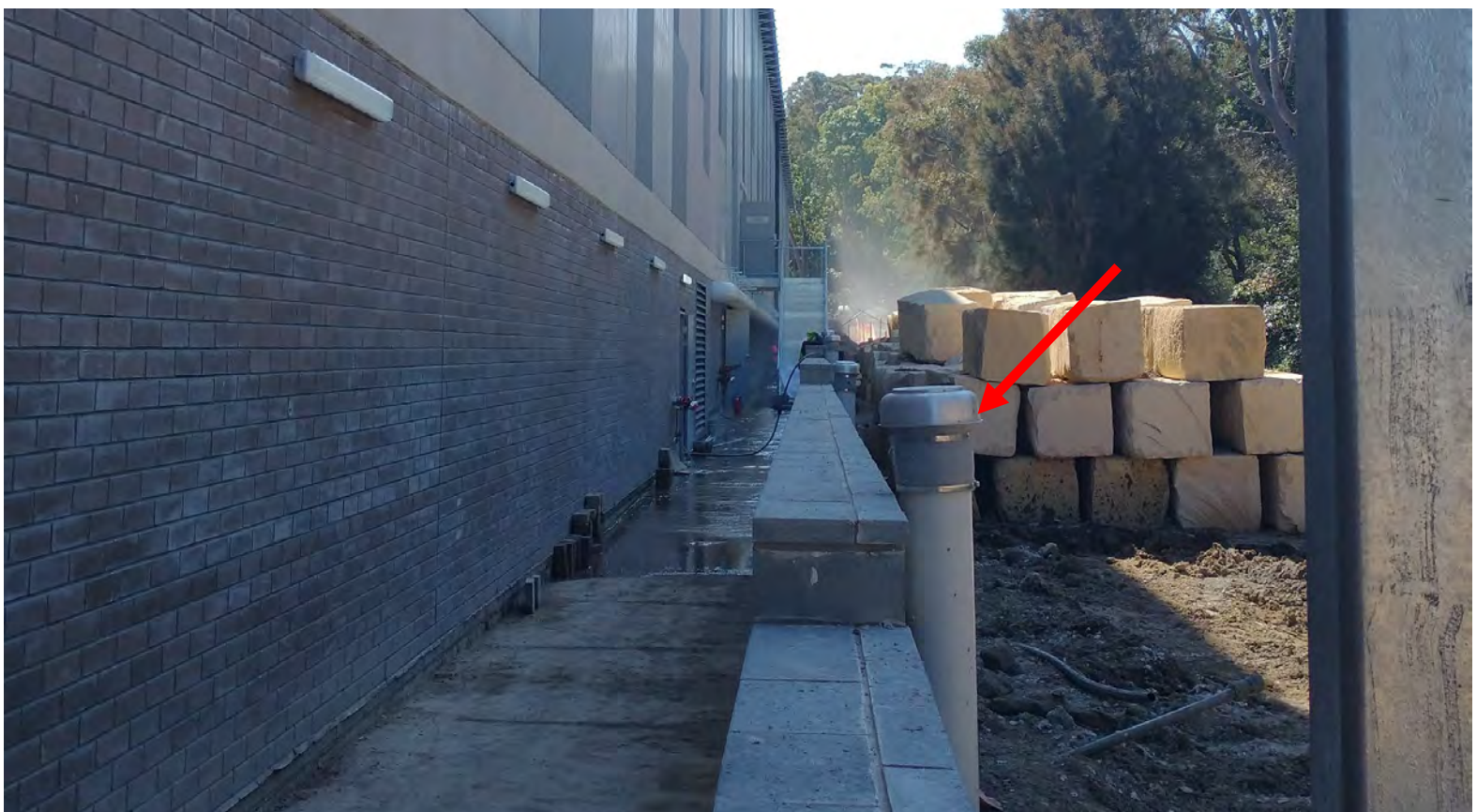
Photograph 5 (facing north): View of a typical 'mushroom cap' inlet pipe (red arrow) east of SSA#1. 11 caps are located along the eastern side of SSA#1.
