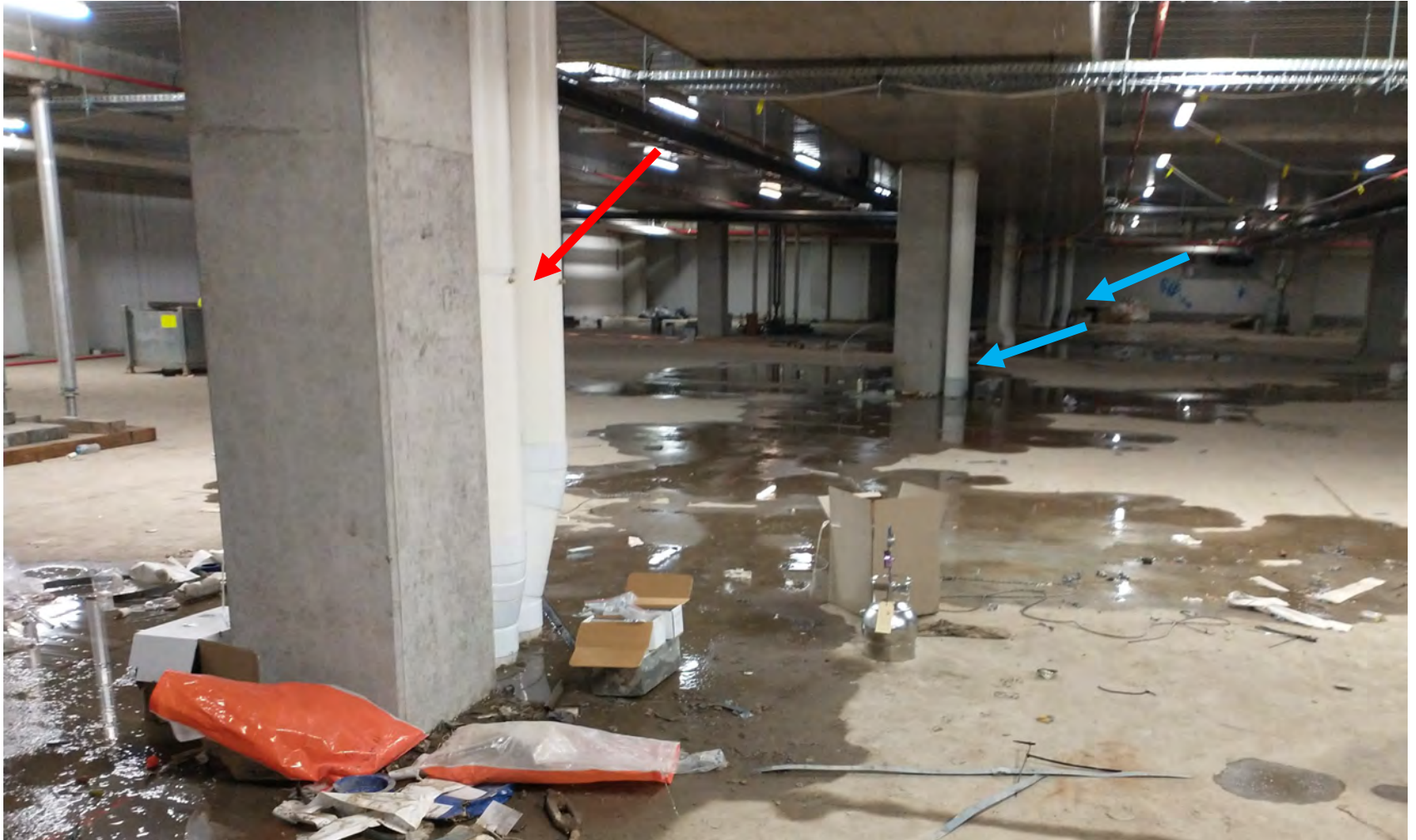
Photograph 6: View of typical outlet risers at SSA#1. Note brass riser sampling ports (red arrow). Additional outlet risers visible in the background (blue arrows).
