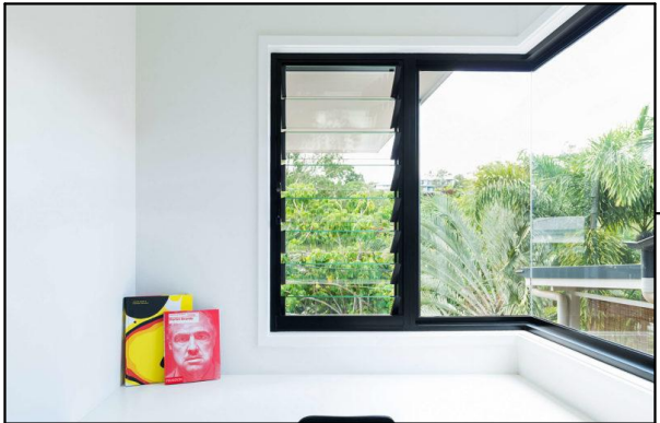
ALUMINIUM FRAMED CORNER WINDOW BY STEGBAR OR OTHER
