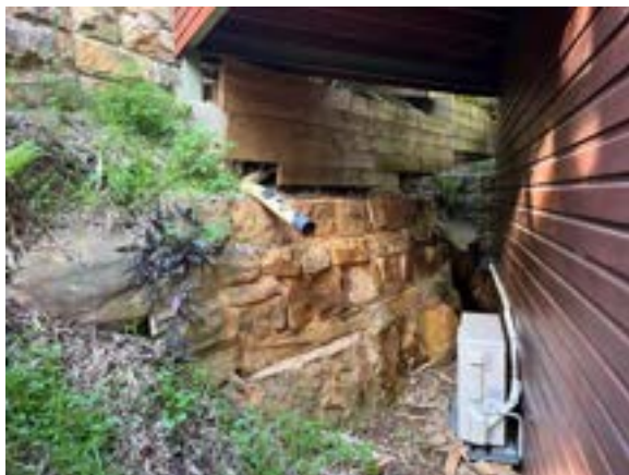
Photo 3: Wall structures at residence frontage and outcropping sandstone bedrock
