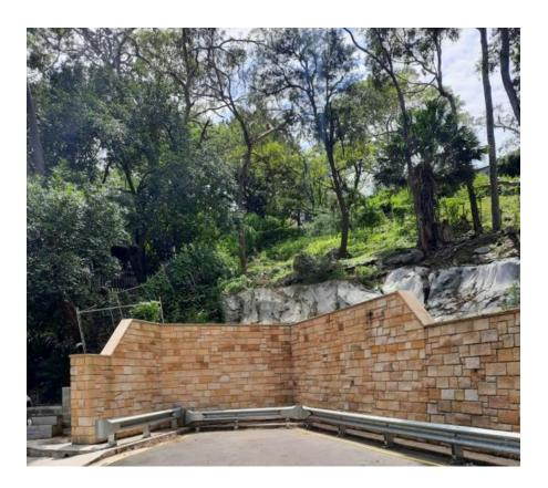
Photo 2 depicts the head of the cul de sac at Bellara Avenue with a 3 plus metre high retaining wall in the mid ground and covered but unsealed deeper excavation behind the wall. The photo is looking north across 32 Bellara Avenue towards the boundary with proposed lot 2.
