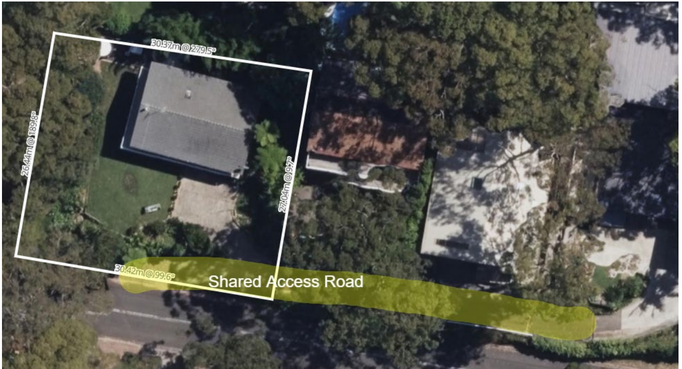
Figure 2: Site aerial (Source: Landchecker)
