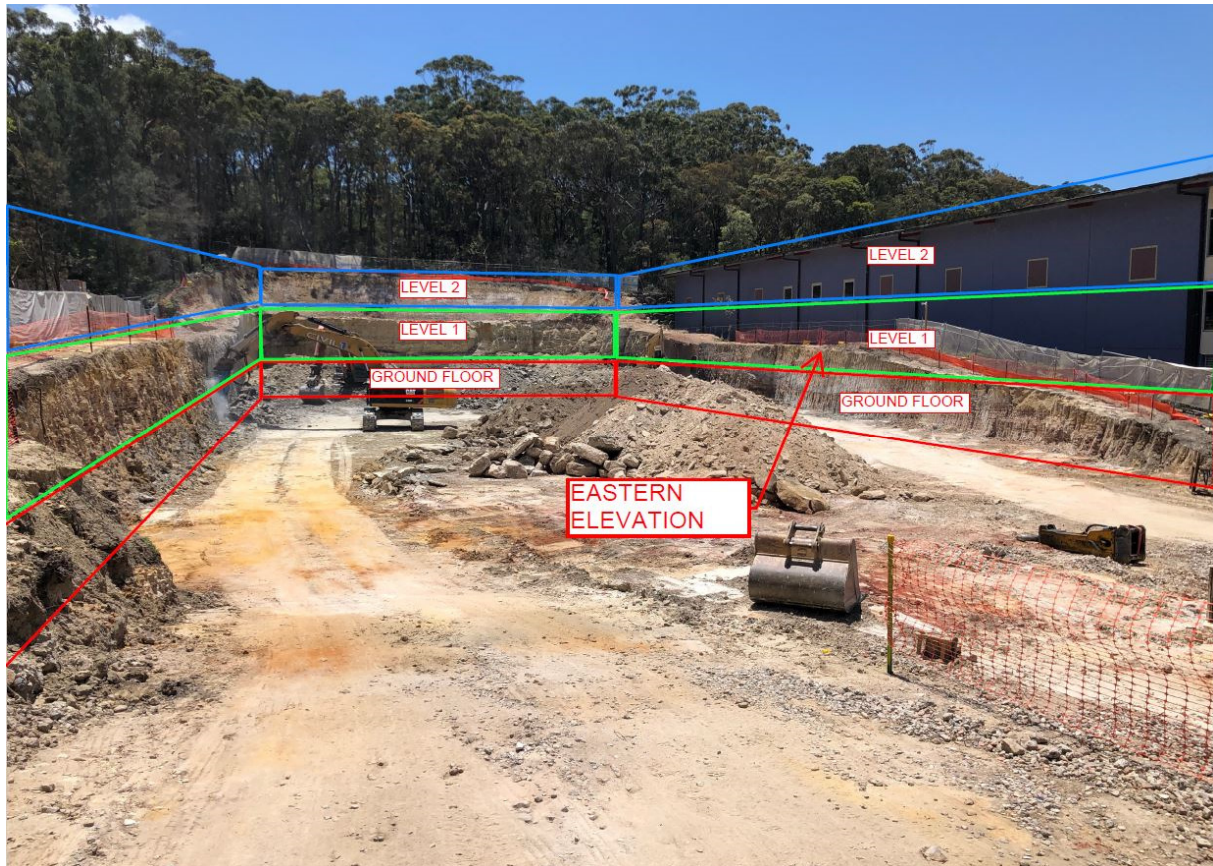
Figure 1: Shielding opportunities offered by earthworks/ retaining walls.
