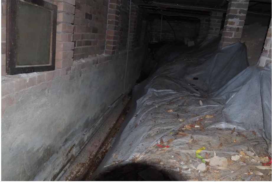
Photo 3: Batter slope below residence covered with geo-fabric
