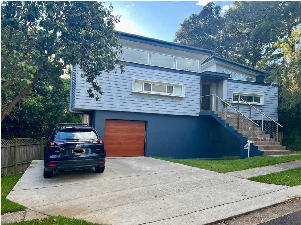
Existing Front dwelling façade (view from streetscape).
