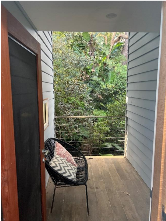
Existing First Floor open reflection area (viewing north)
