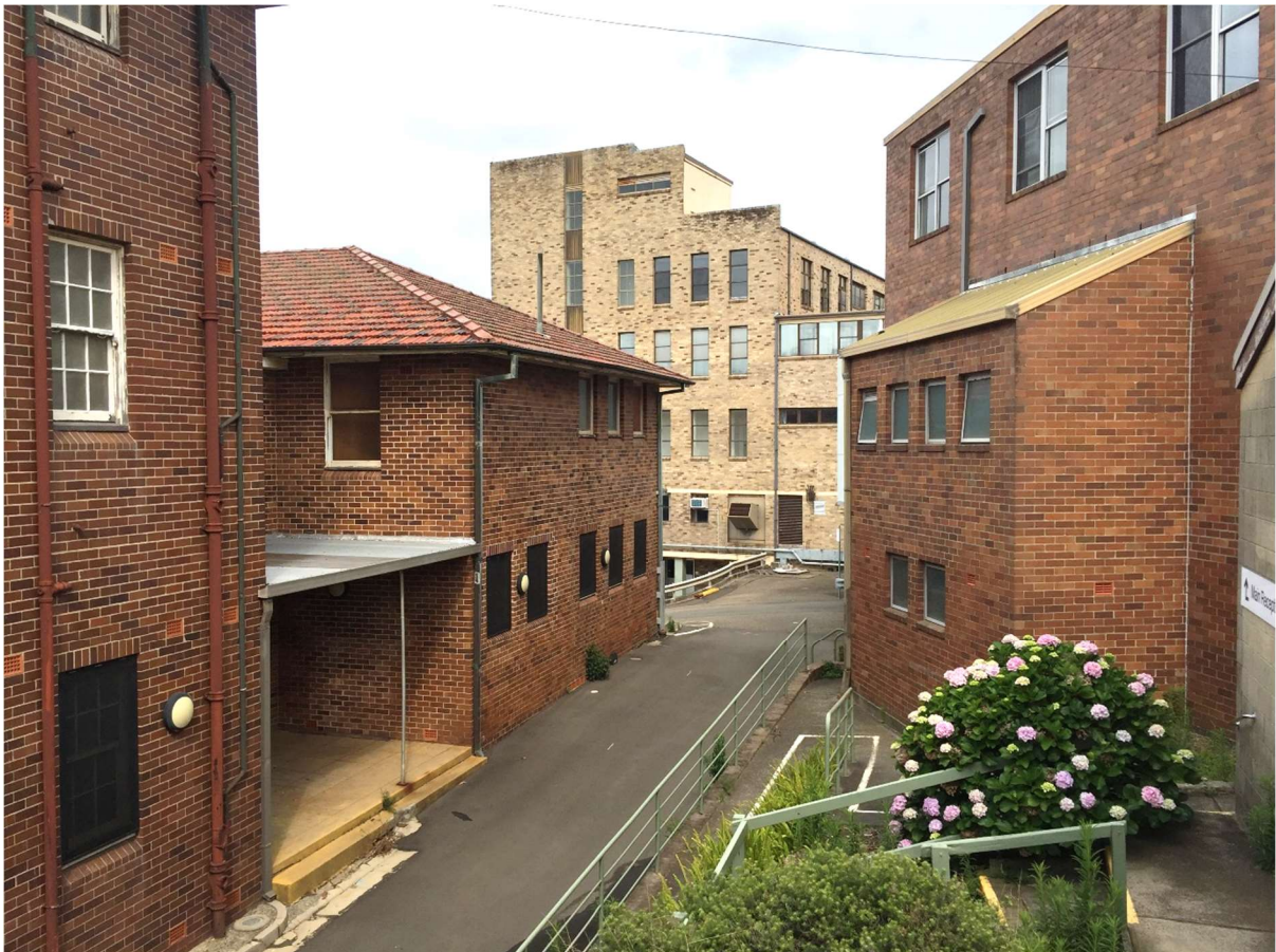
Photo 2: Internal Roadway – Rear of Existing Hospital Main Building
