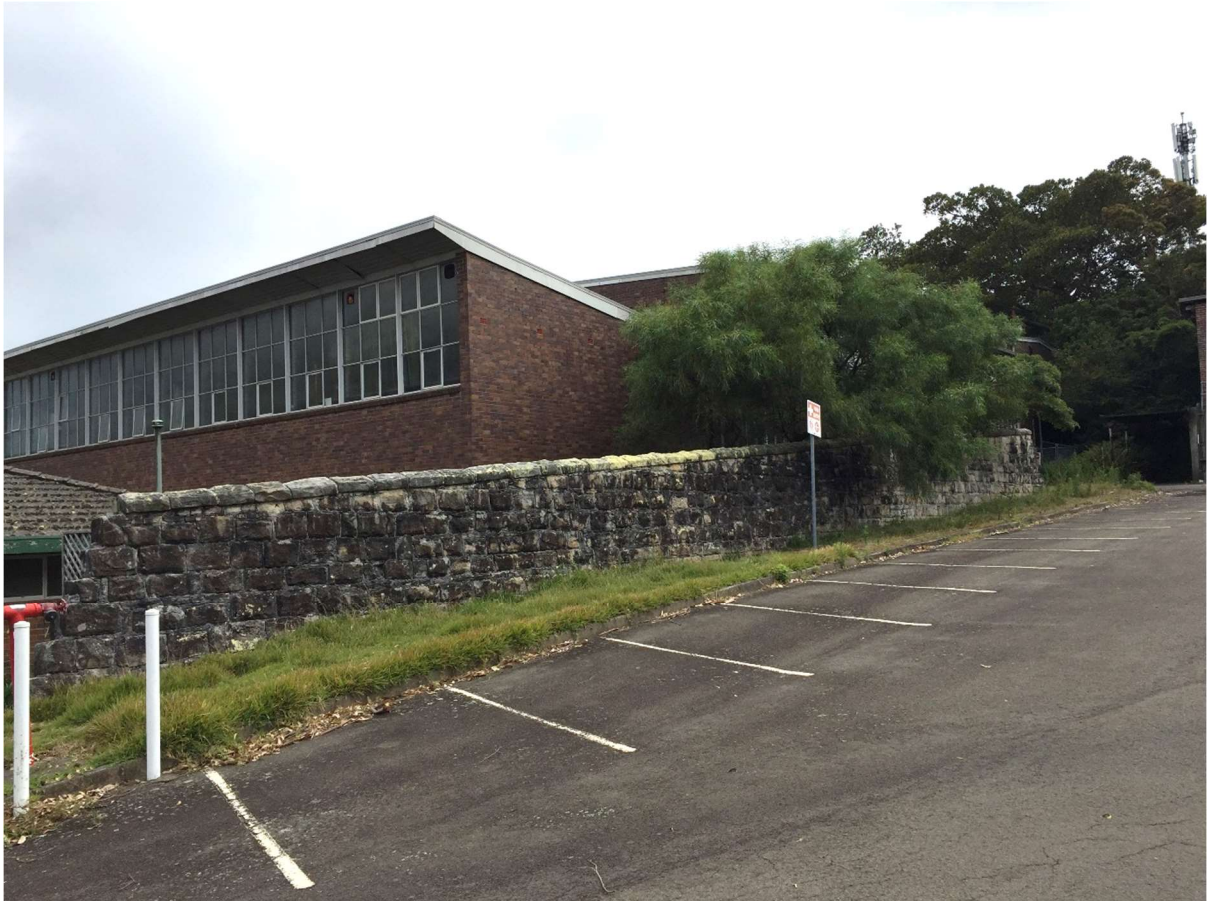
Photo 8: Sandstone Wall Parallel to Stormwater Trunk Drainage Line
