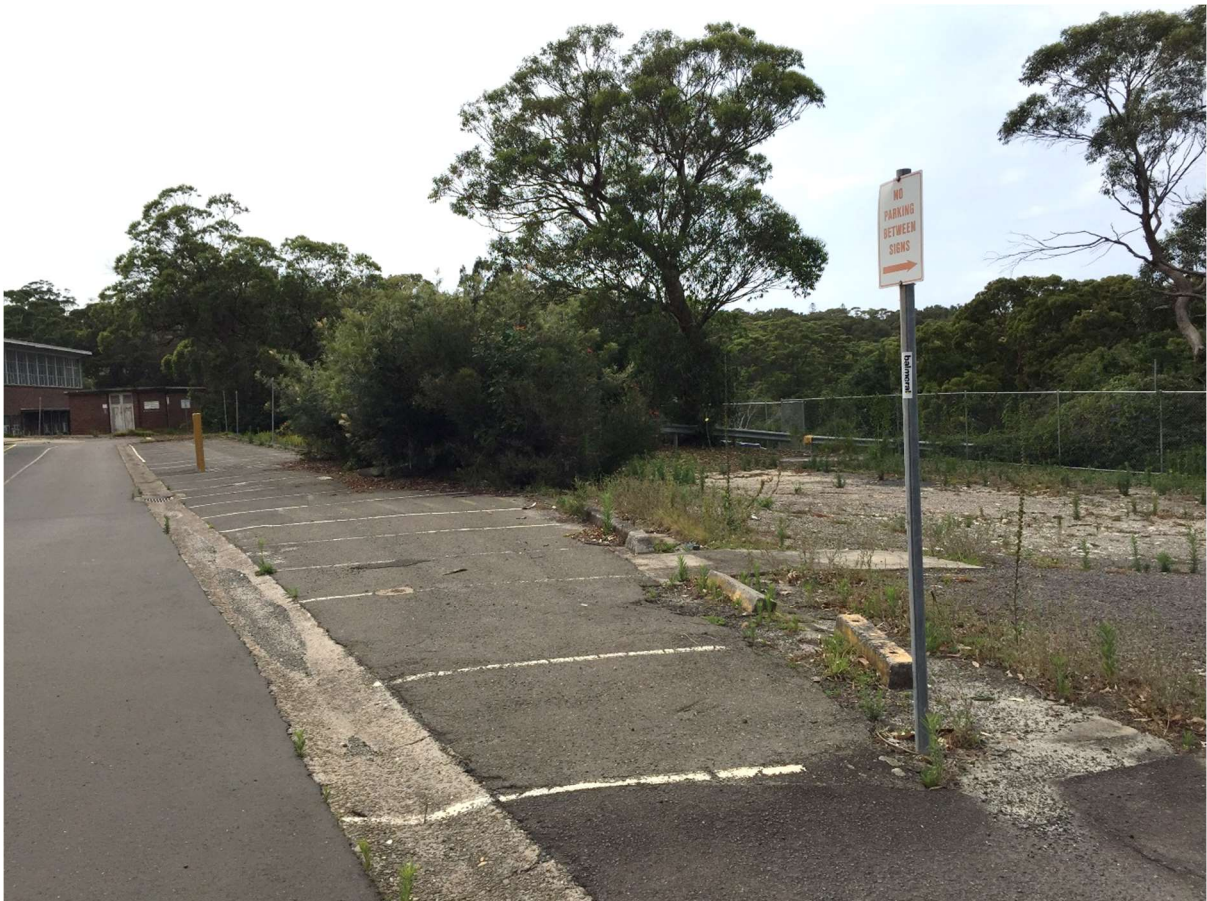
Photo 4: Internal Roadway and Southern Carpark with Dish Drain
