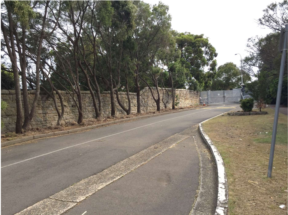
Photo 3: Internal Roadway – Approach to Darley Road from Southern Carpark Areas
