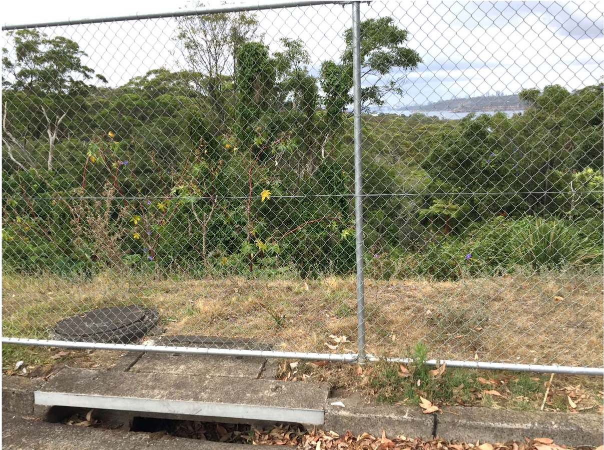
Photo 6: Kerb Inlet Pit and Dense Bushland along Southwest Boundary of Lot 2619
