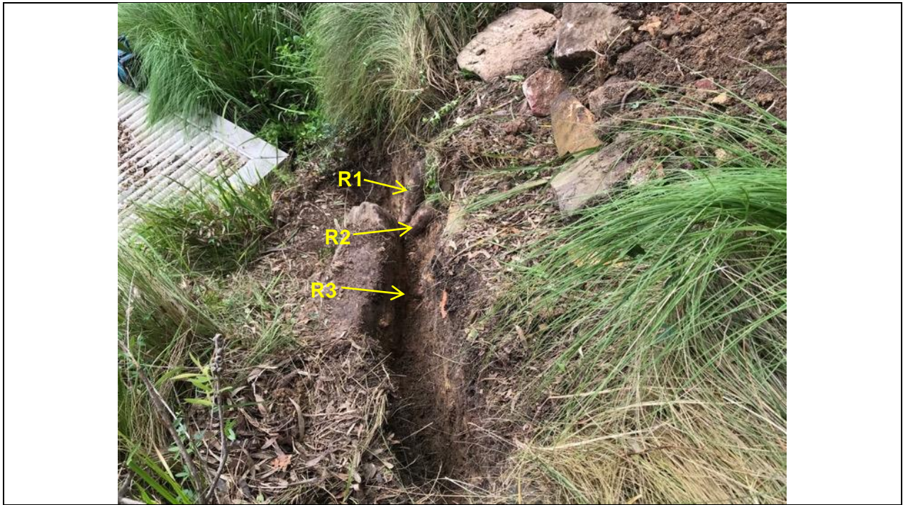
Image 3: Looking North East along root investigation trench 1. Showing location of root 1, 2 and 3.
