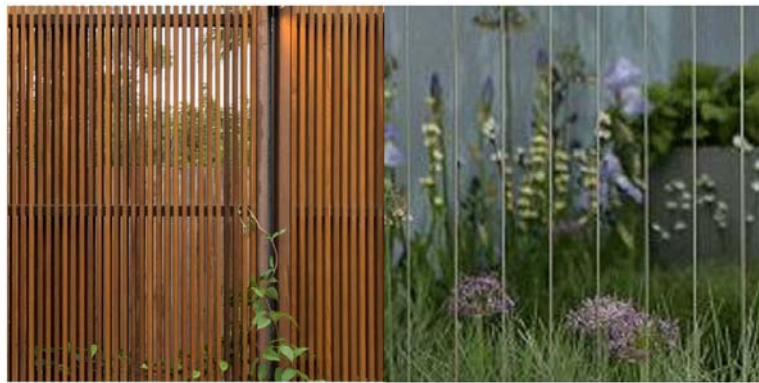
7 TIMBER BATTENS AND STEEL CABLE WIRES
