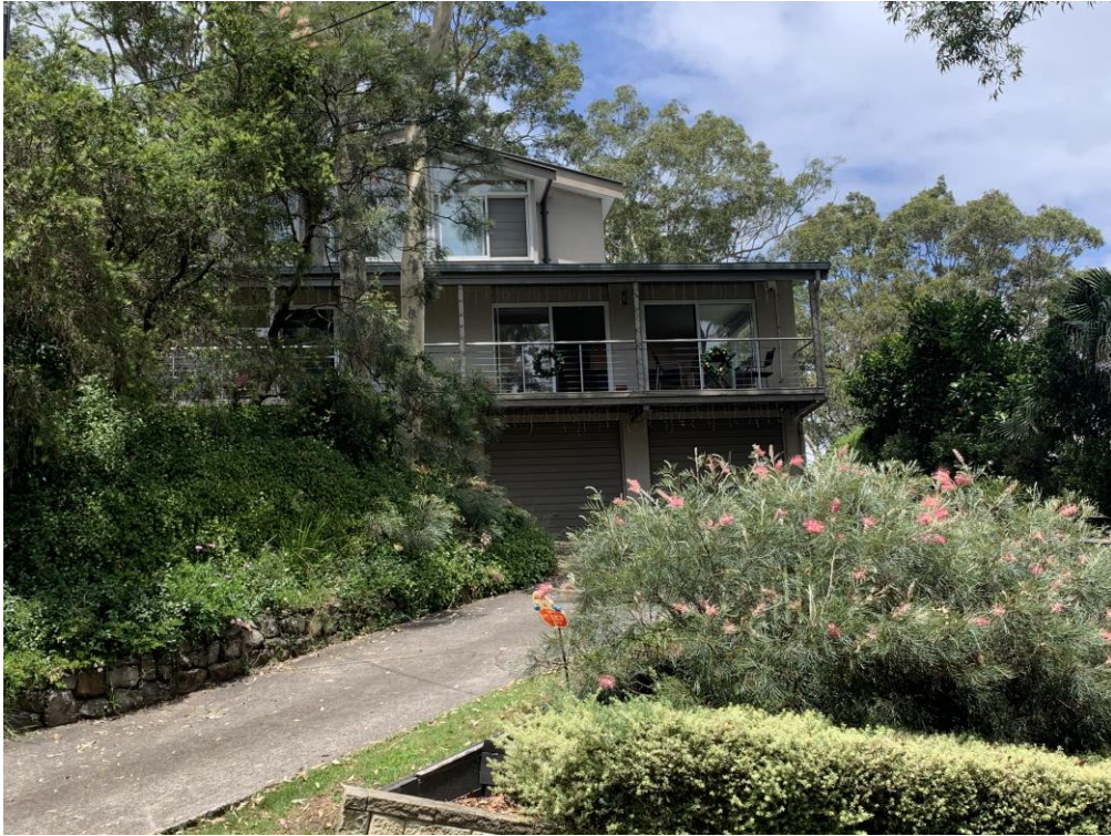
Fig 2: View of subject dwelling, looking south from Wandeen Road
