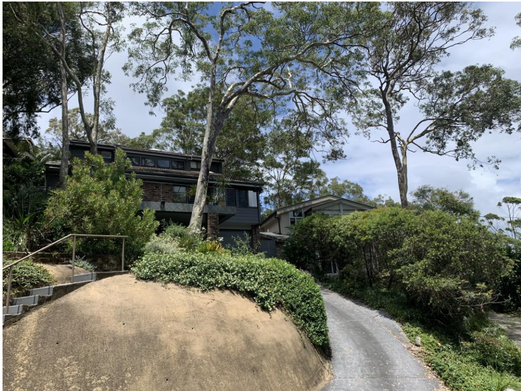
Fig 5: View looking towards the subject site and the neighbouring dwelling at No 31 Wandeen Road, looking south-west from Wandeen Road
