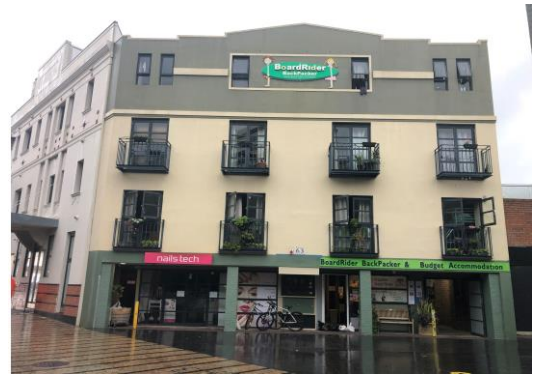
Figure 5: Subject site from rear, Market Place.
