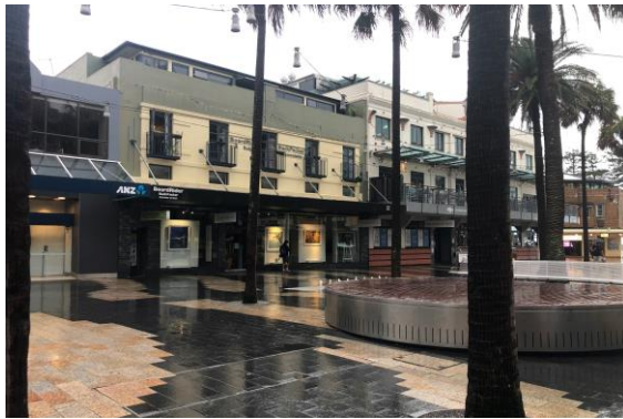
Figure 4: Subject site with The Corso street frontage, with neighbouring properties in sight
