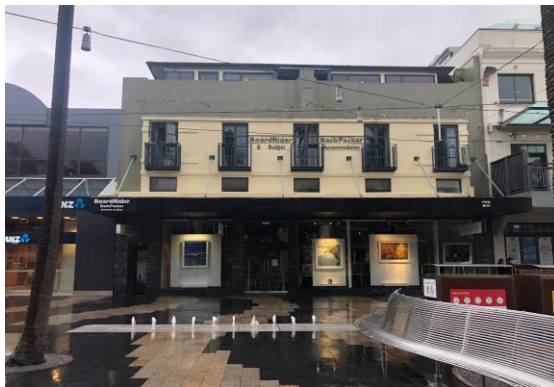
Figure 6: Subject site from the Corso
