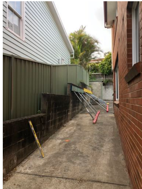
Figure 3, View of existing dilapidated retaining wall.
