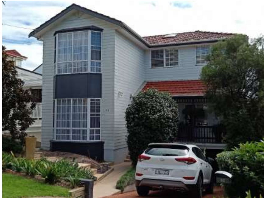
Photo 1: View of existing dwelling from Innes Road also showing the existing two storey bay window to be removed and replaced with the first floor deck and the front windows to be replaced with new windows to fit within the existing window opening.
