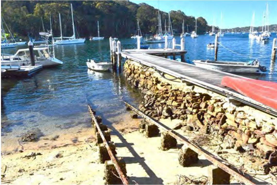
Figure 3 View of western side of facility showing sliprails, stone jetty with wood deck and offshore jetty.
