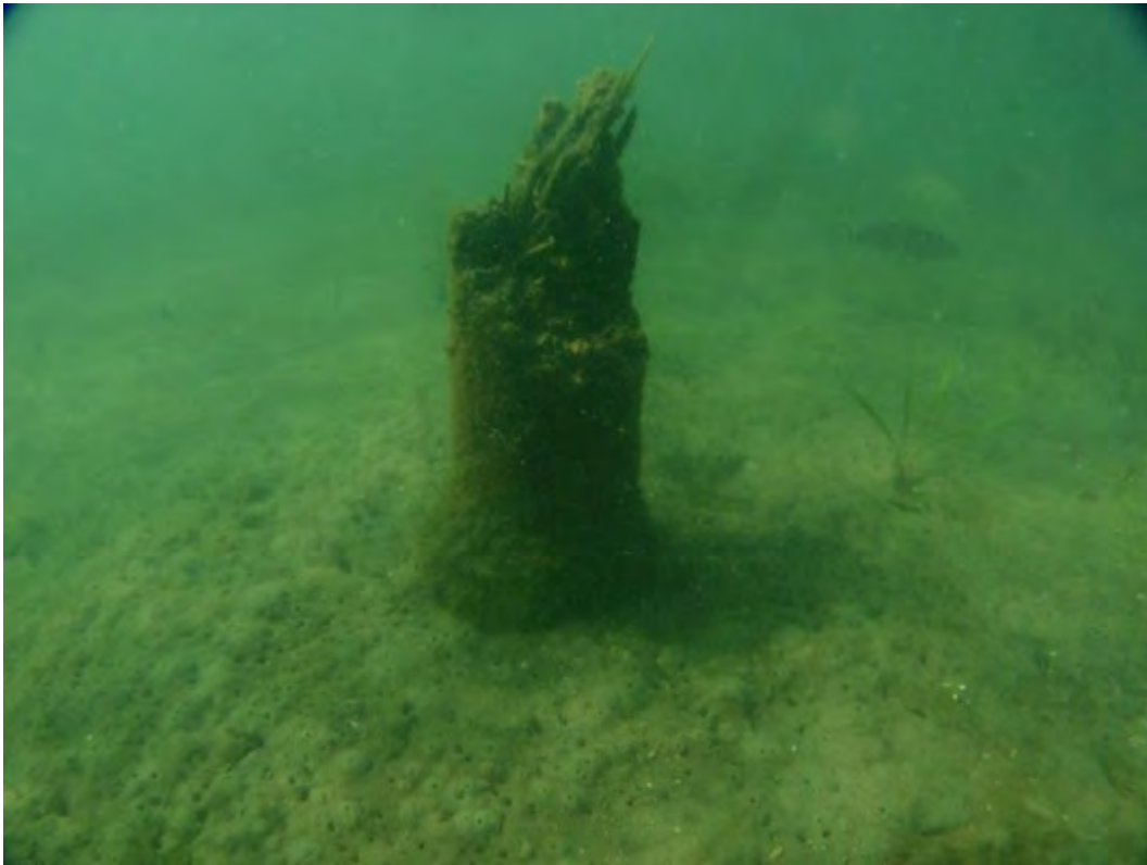
Figure 13 Outer snapped off mooring pile with very sparse Posidonia cover in vicinity.
