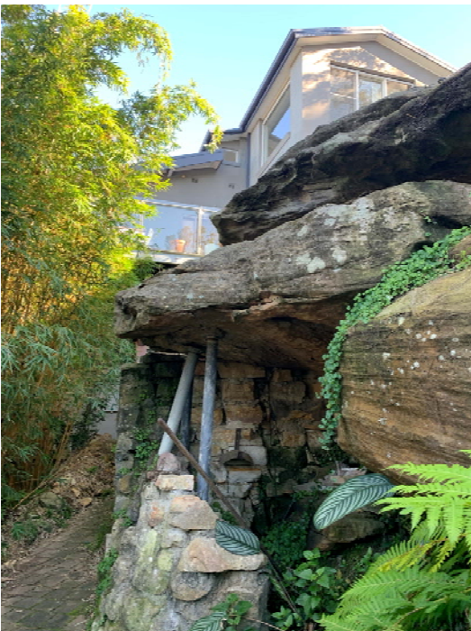
Existing undercut cliff face showing supporting posts
