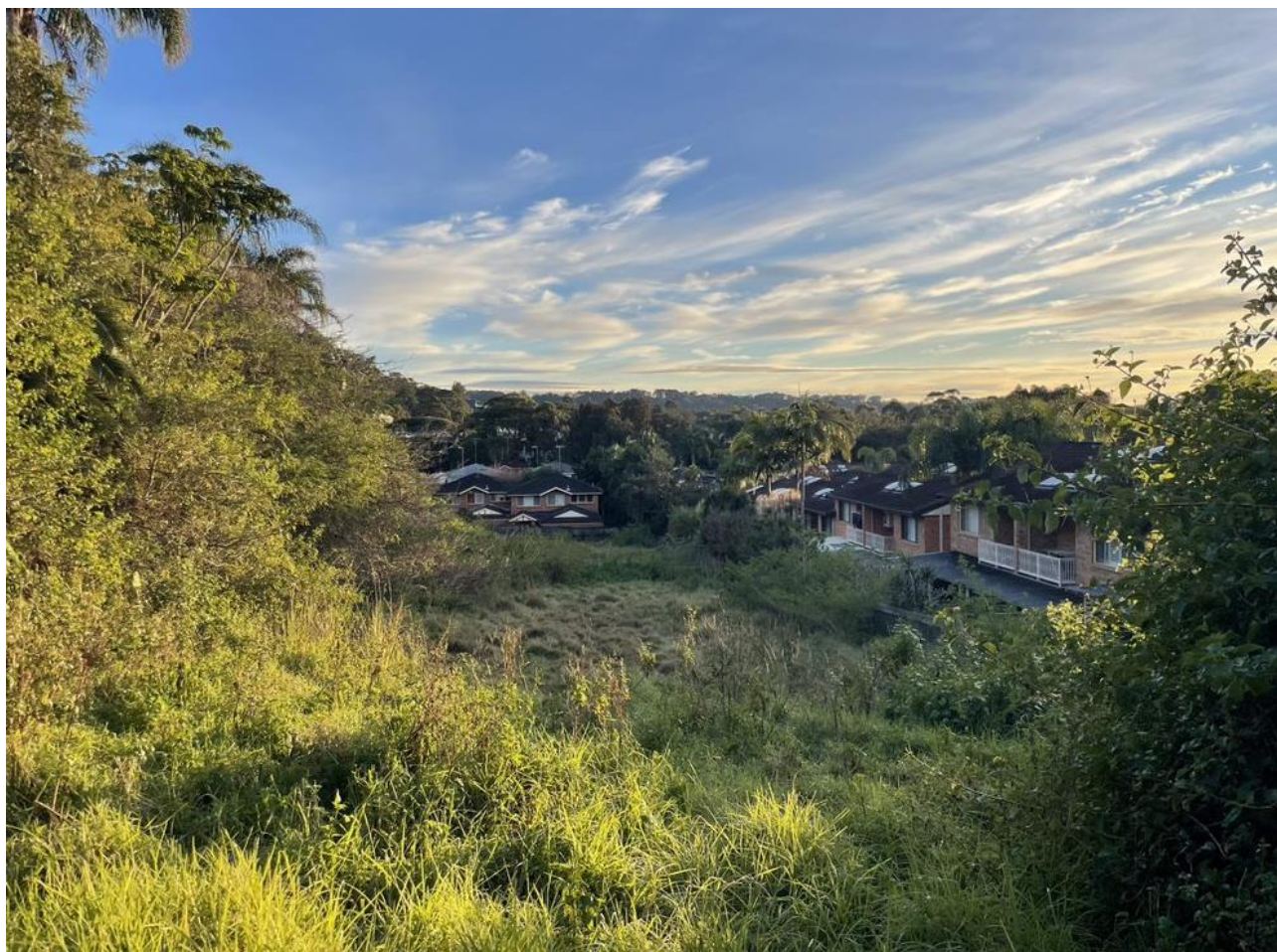
Photo 2: Looking North-east from the driveway toward the lower elevations of the subject site.
