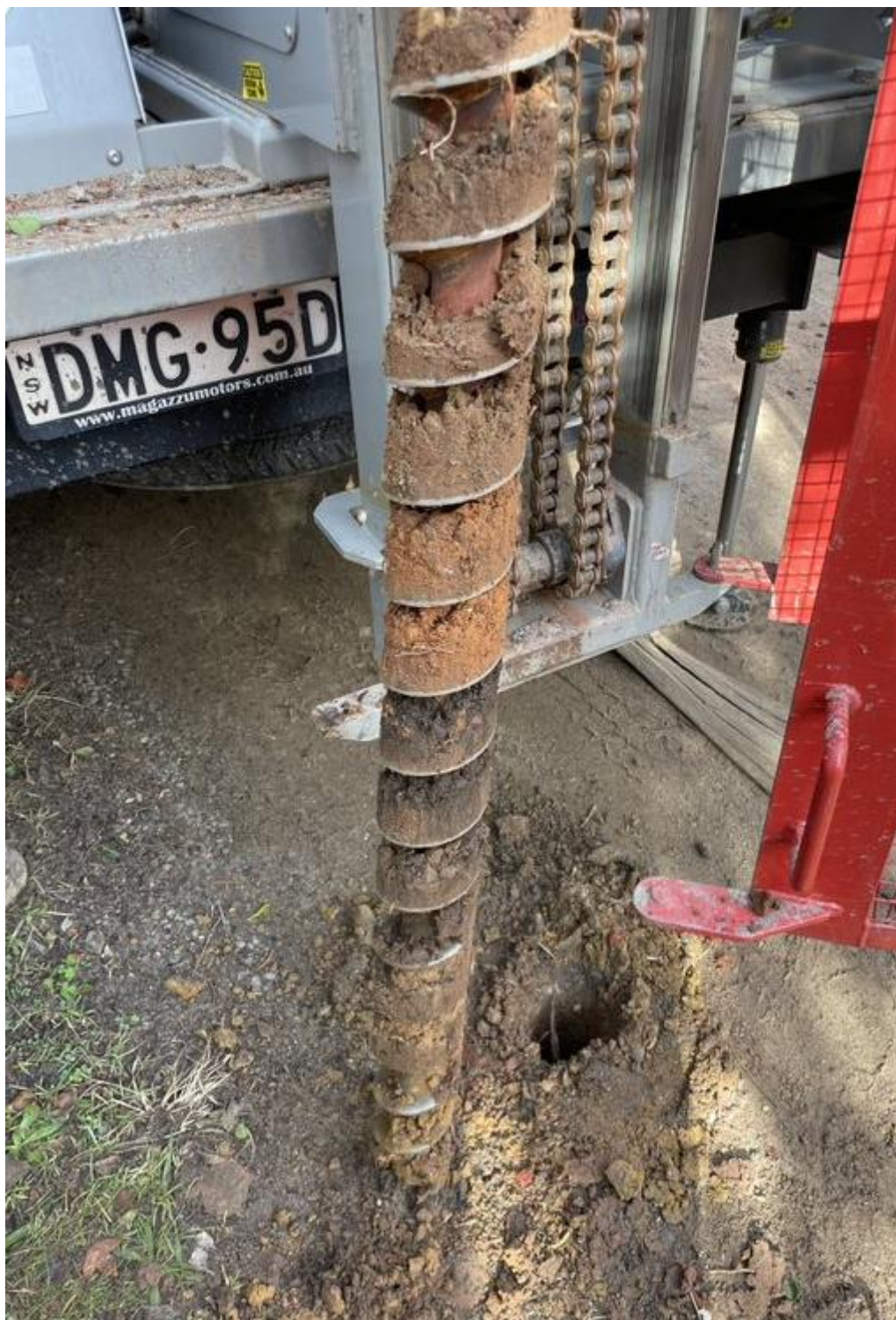
Photo 3: Fill materials on the auger from BH101
