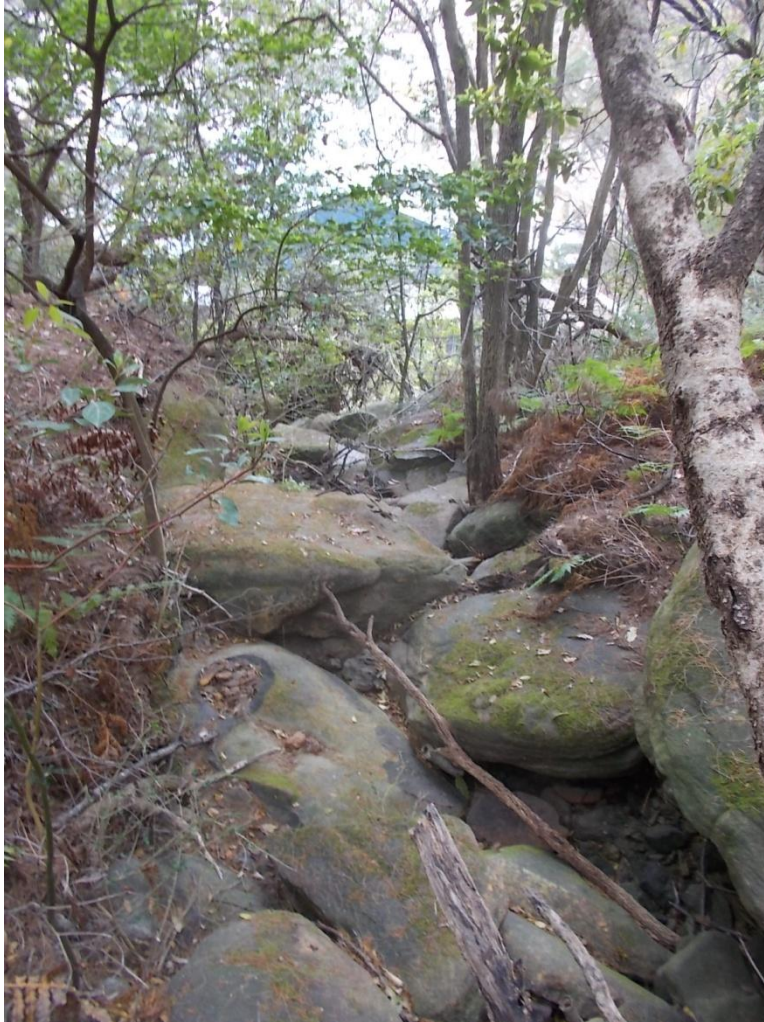
Figure 9 - Small rock-lined drainage channel flowing eastwards down the slope to established piped stormwater infrastructure below cliffline
