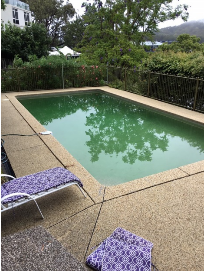
Figure 2 Image of the existing pool on site
