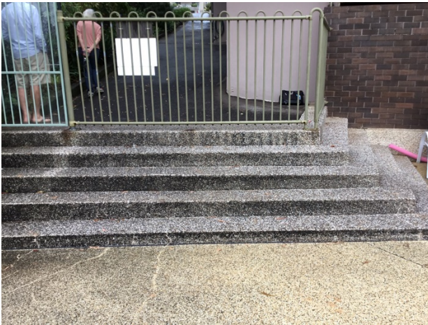
Figure 5 Existing steps into the pool area
