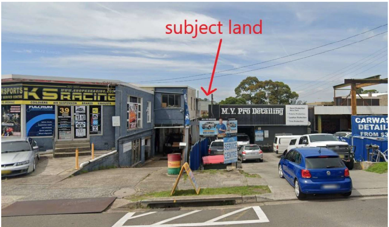
Figure 3 Streetview (subject site runs between the two buildings pictured)
