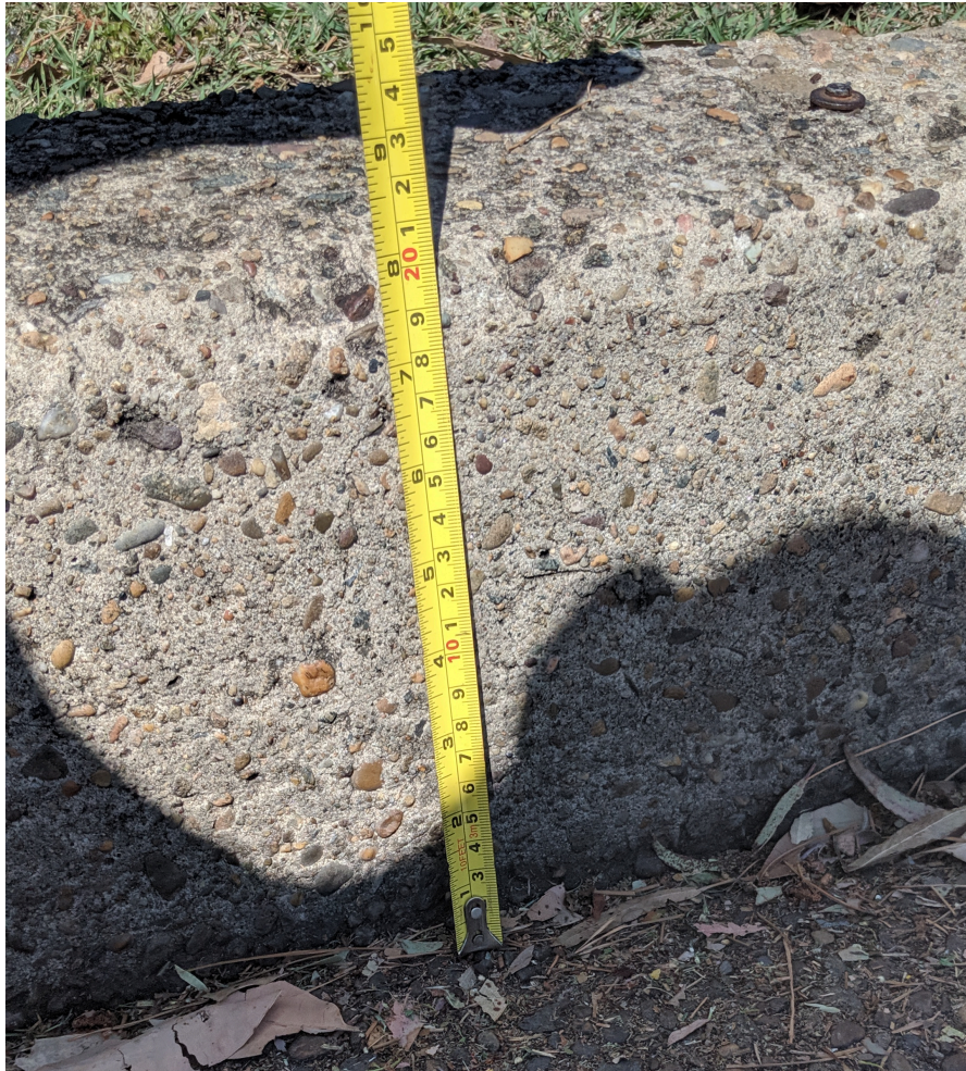
Image 1 - Kerb height, South Creek Road (south alignment)
