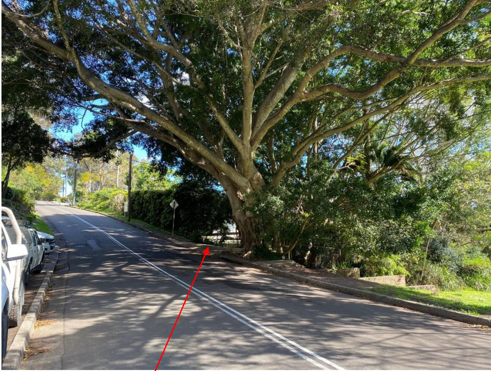
Photograph of the existing driveway entrance to the site
