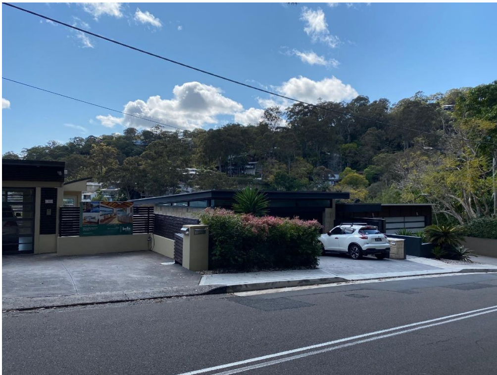
Photograph of adjoining properties to the west along Prince Alfred Parade - # Note the structures above the road and front setbacks provided
