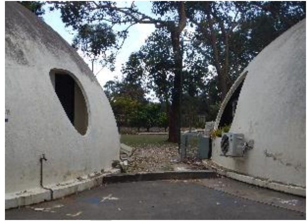
FIGURE 3.23: EXTERNAL UNIT ATTACHED TO SHELL AND ADDITIONAL SERVICE PENETRATIONS LOW TO THE GROUND.
