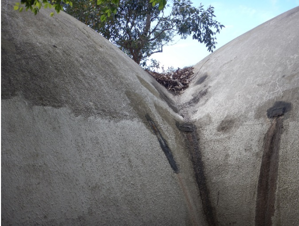
FIGURE 3.18: PATCHING OF MEMBRANE AROUND INTERSECTION OF DOMES, BINISHELL B. NOTE ALSO BUILD-UP OF PLAT DEBRIS.
