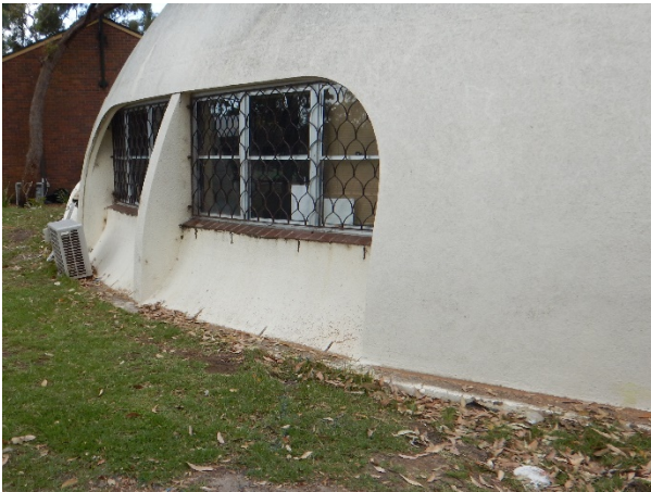
FIGURE 3.20: EXAMPLE OF GROUND BUILT UP AROUND THE BASE OF THE BINISHELLS. NOTE RING BEAM ONLY PARTIALLY EXPOSED ON THE RIGHT, BUT LARGELY COVERED ON THE LEFT.
