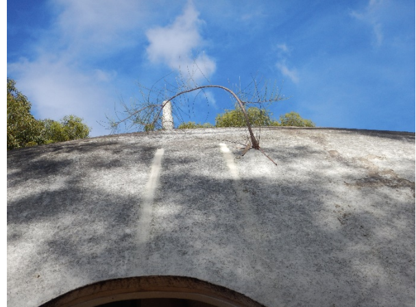
FIGURE 3.19: PLANT GROWING FROM MEMBRANE AND SHELL OF BINISHELL A.
