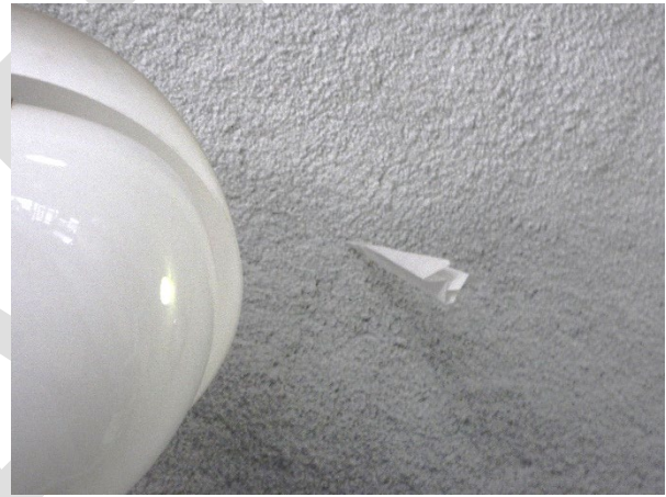
FIGURE 3.21: SPRAY VERMICULITE CEILING IS FLAKY, CREATING A DUST HAZARD. EMBEDDED PAPER PLAN DEMONSTRATES HOW SOFT THE INSULATION LAYER IS.
