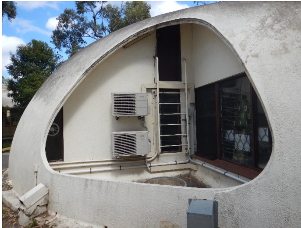
FIGURE 3.22: EXAMPLE OF EXTERNAL SERVICE ADDITIONS WITHIN BINISHELL OPENINGS AND SECURITY SCREEN TO WINDOW.
