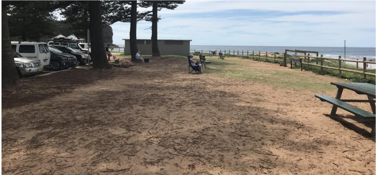
Figure 3: View of existing amenities building from reserve to SW, looking ENE
