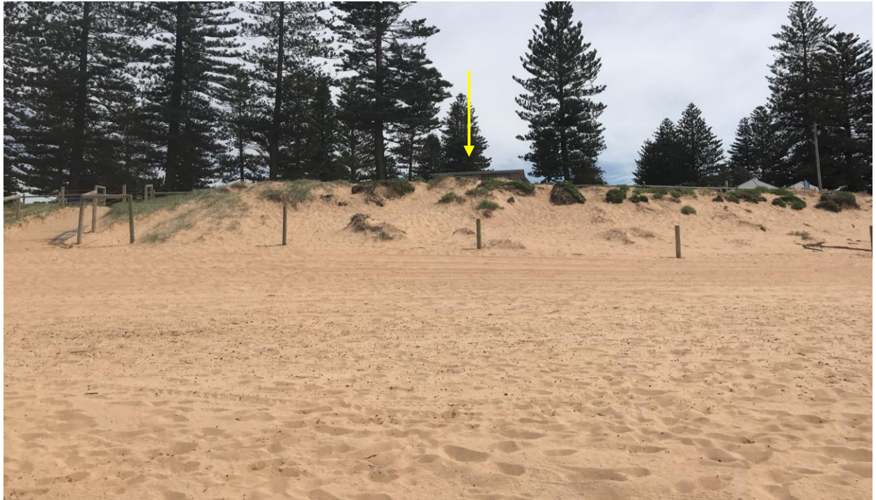
Figure 1: View of existing amenities building (at arrow) from Mona Vale Beach, looking NNW
