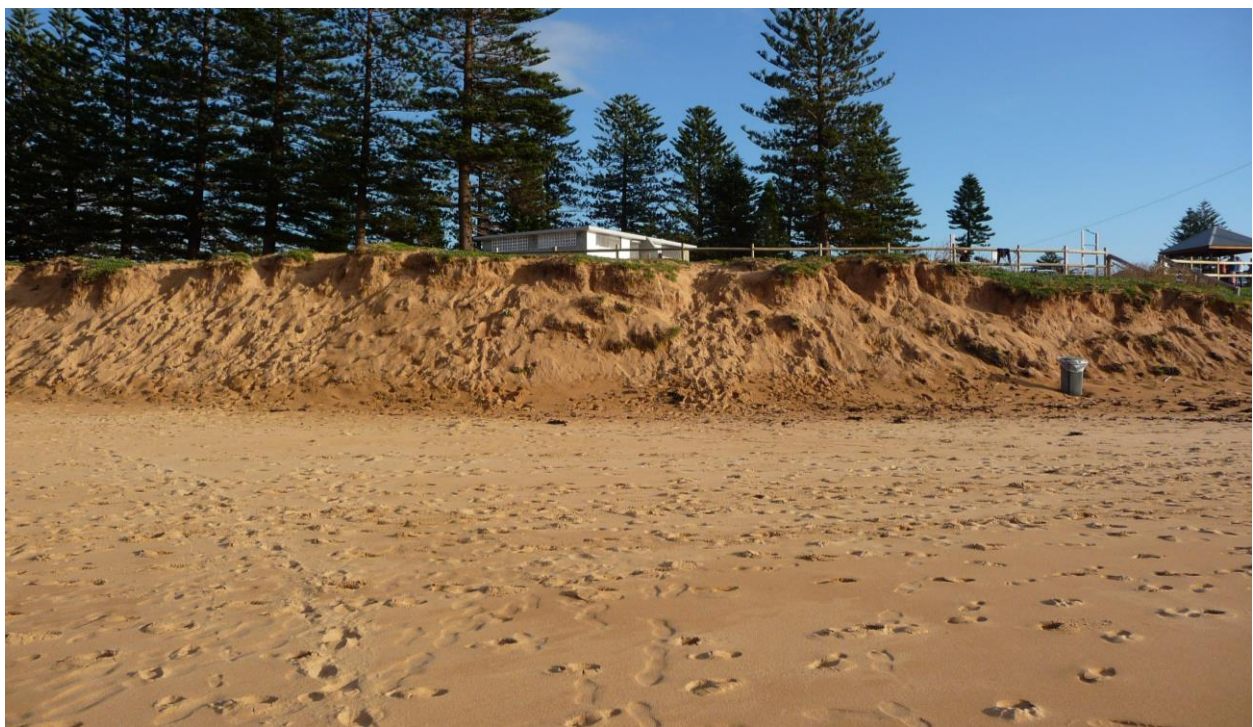
Figure 4: Erosion seaward of amenities building evident on 6 June 2015
