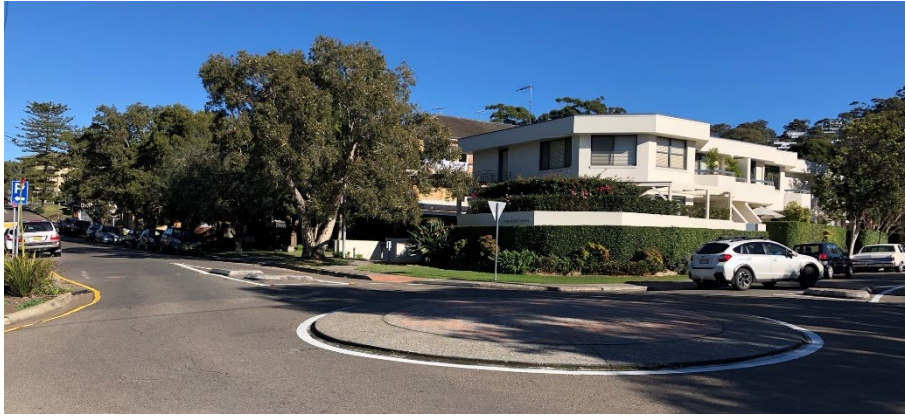
Photograph 12: View of Newport Anglican Church, located to the north of the site at the boundary interface
