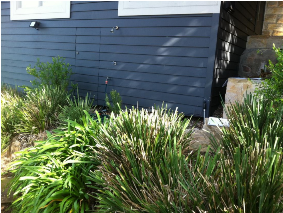
Image 2 - View west towards residence, showing proposed location of spa and access door to undercroft area.
