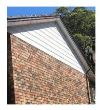
New walls - BRICKS AND WEATHERBOARD - TO MATCH EXISTING
