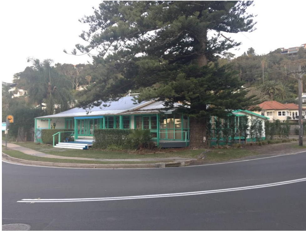
Fig 2: View of subject site as viewed from Barrenjoey Road/Beach Road intersection, looking south-east
