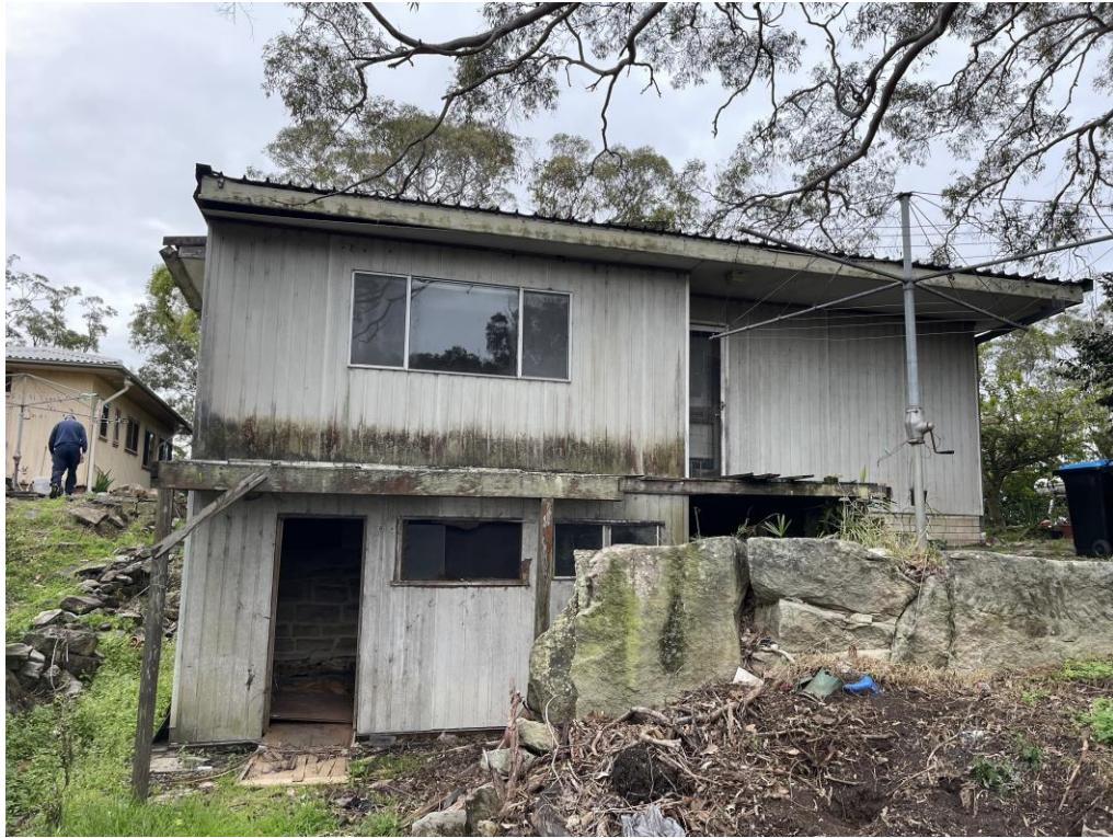
Fig 9: View of the southern (rear) elevation of the dwelling, looking north
