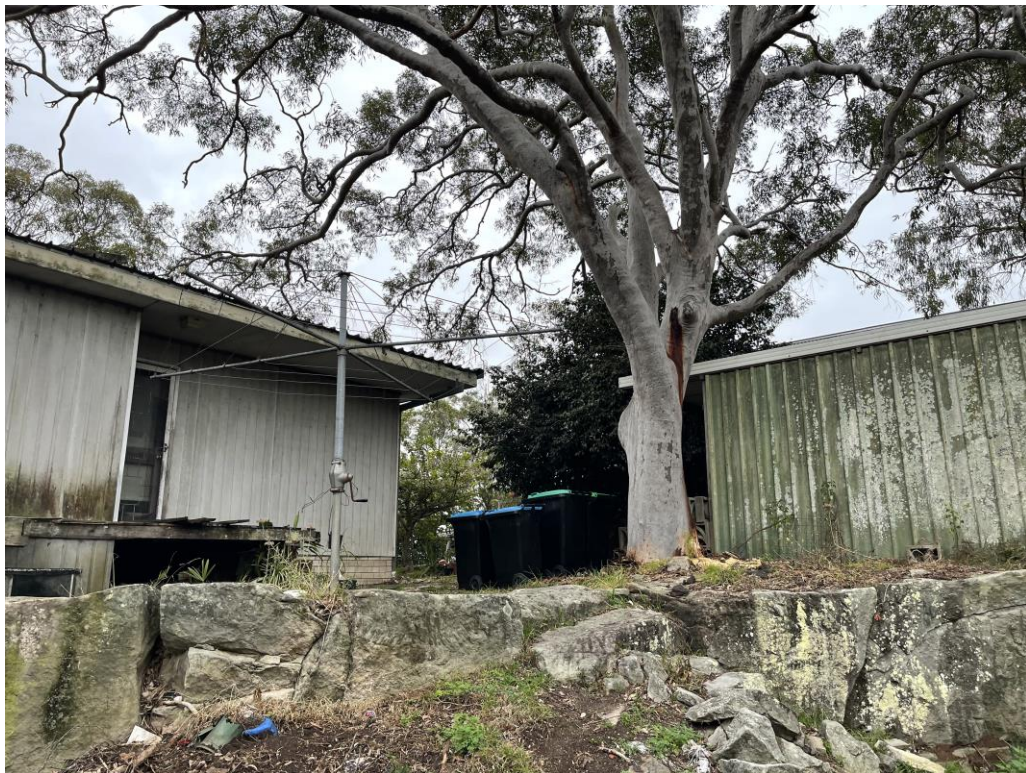
Fig 10: View of the existing dwelling and detached carport, looking north-east
