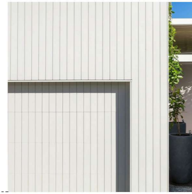
FC - FIBRE CEMENT CLADDING - JAMES HARDIE 'AXON' 133MM SMOOTH PAINTED 'OFF WHITE'
