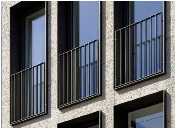
BAL 1 ALUMINIUM - BALUSTRADE, FINISH SIM/EQ TO DULUX POWDERCOAT 'MONUMENT'
