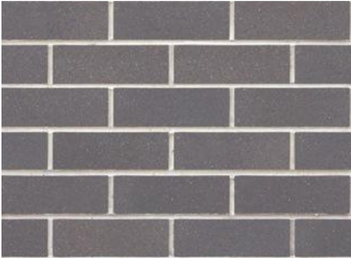
FBK 1 FACE BRICKWORK FINISH - AUSTRAL BOWRAL BRICKS 'BRAHMAN GRANITE'
