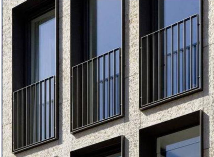
ALU 1 ALUMINIUM - WINDOW/BALCONY SURROUNDS, FINISH SIM/EQ TO DULUX POWDERCOAT 'MONUMENT'
