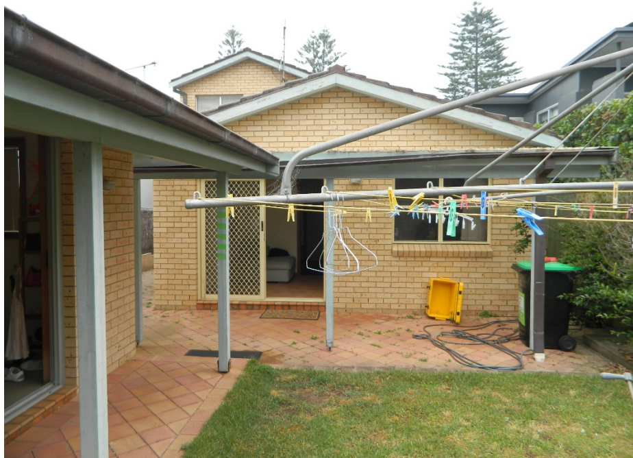
Photograph 2: The rear façade of the existing dwelling house on the subject site.
