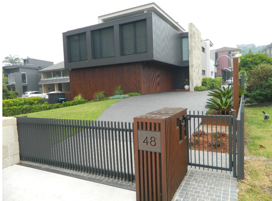
Photograph 5: The recently constructed dual occupancy 20m to the south-east of the site, 48 Kooloora Avenue.
