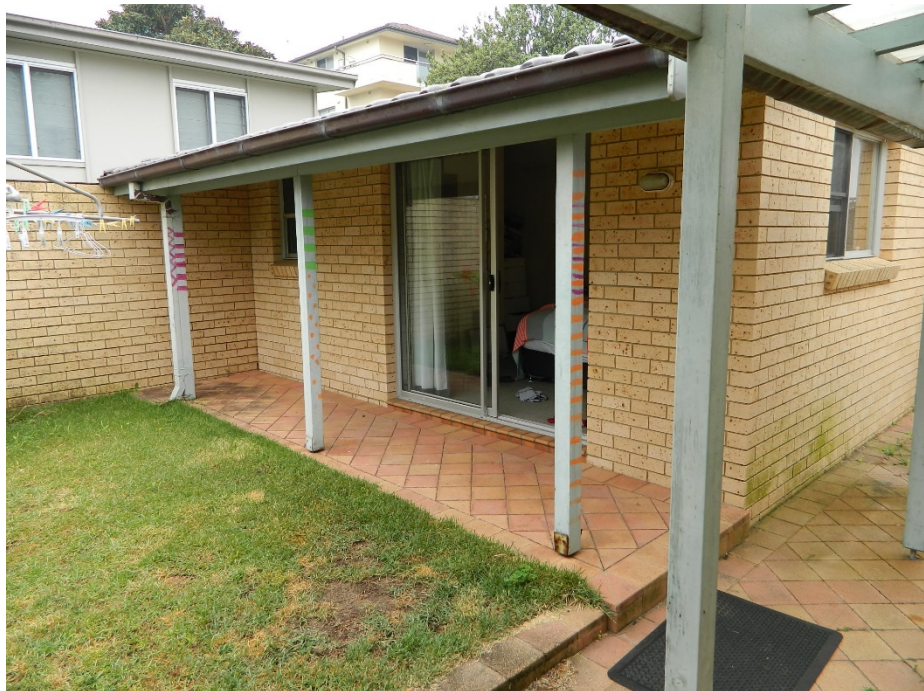
Photograph 3: The existing outbuilding in the rear yard on the subject site.
