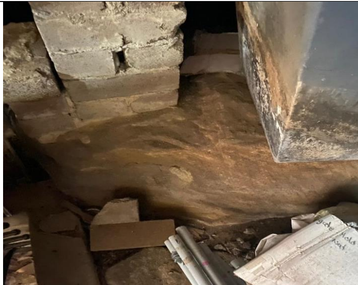
Photo 3: Exposed sandstone bedrock supporting brick pad footing of the existing dwelling.
