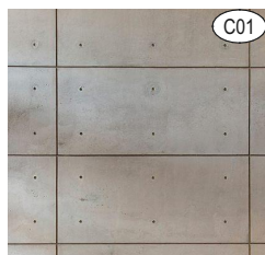
OFF FORM CONCRETE
