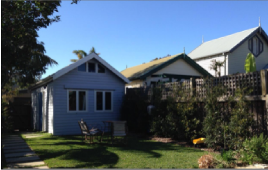
View of Existing Carport from yard
