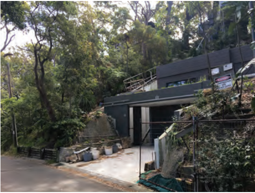
Plate 5: View looking west along Chisholm Avenue. The garage building sits at the base of No. 52 Chisholm Avenue and the boundary of No. 52 and No. 60 sits just beyond the building. This garage has a substantial impact on the surrounding bushland setting.
