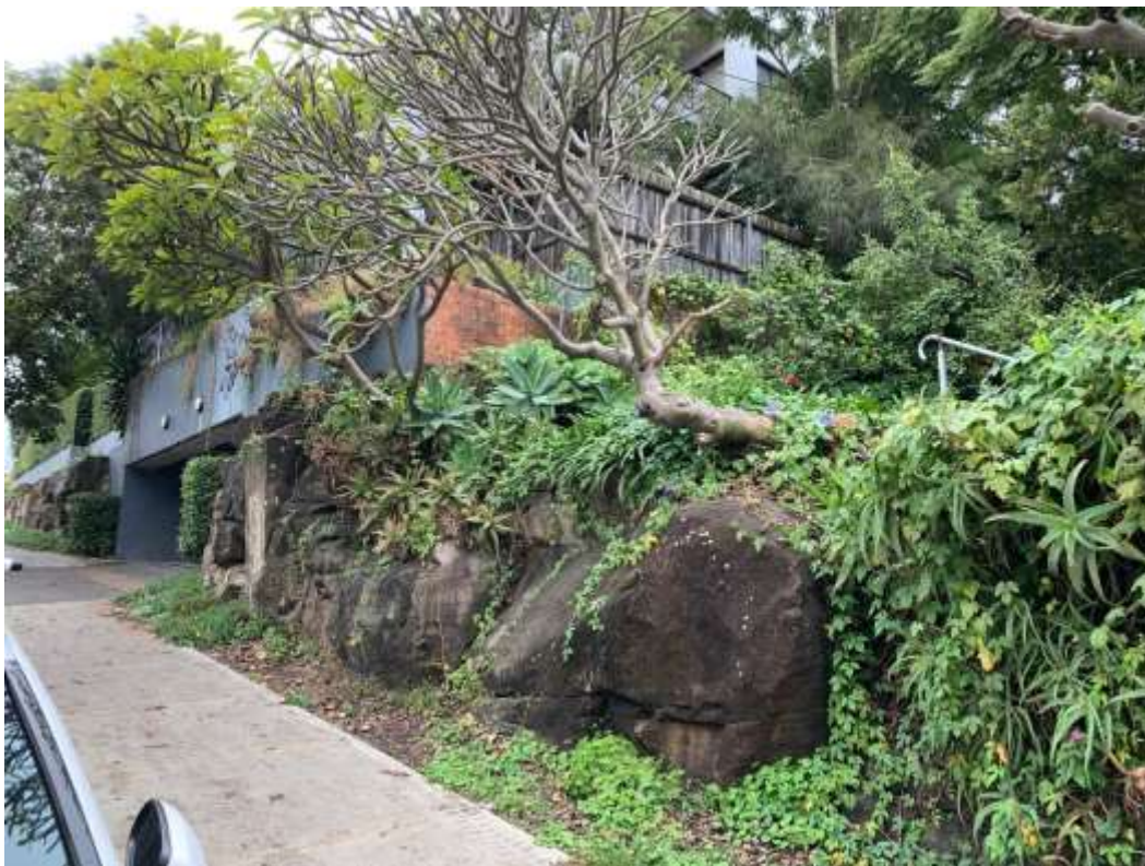
Figure 2: Unsupported rock wall at the front of the site
