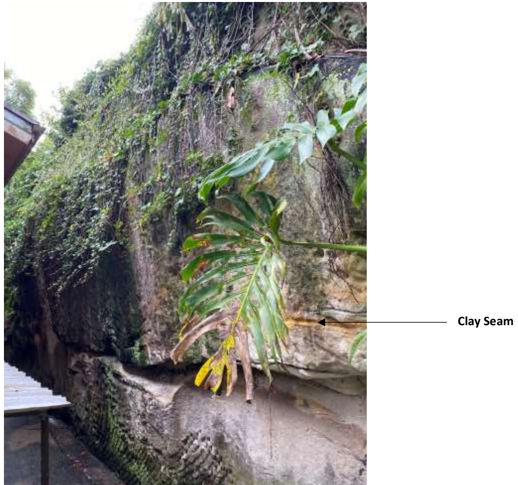
Figure 5: Unsupported sandstone rock at eastern side of the site
